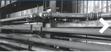
THE PRINCIPAL ADVANTAGE OF RUBBER-LINED STEEL PIPE IS ITS STRUCTURAL CAPACITY REQUIRING NO ADDITIONAL BEAMS FOR INSTALLATION.
