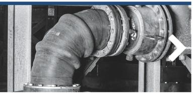
RUBBER BENDS ARE INSTALLED IN PARTS OF A HOSE SYSTEM REQUIRING ELEVATED WEAR RESISTANCE WHERE RUBBER HOSE CANNOT PROVIDE THE REQUIRED BENDING RADIUS. BENDS ARE USED TO CHANGE THE DIRECTION OF ABRASIVE MIXTURE FLOW DURING TRANSPORTATION.
