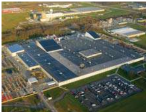
Richmond, KY - Manufacturing Plant
