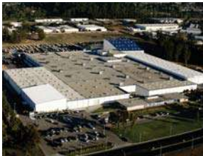
Santa Maria, CA - Manufacturing Plant
