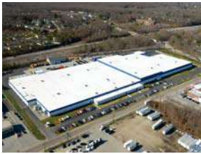
Cumberland, RI - Manufacturing Plant
